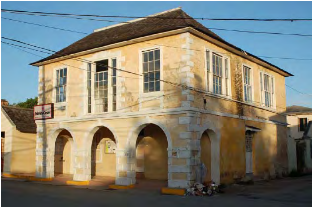
Post Office, Falmouth. Originally constructed in 1832 as a house and store for a British merchant, the building incorporates rendered masonry construction, a covered arcade, and hipped roof in an elegant but compact design.
