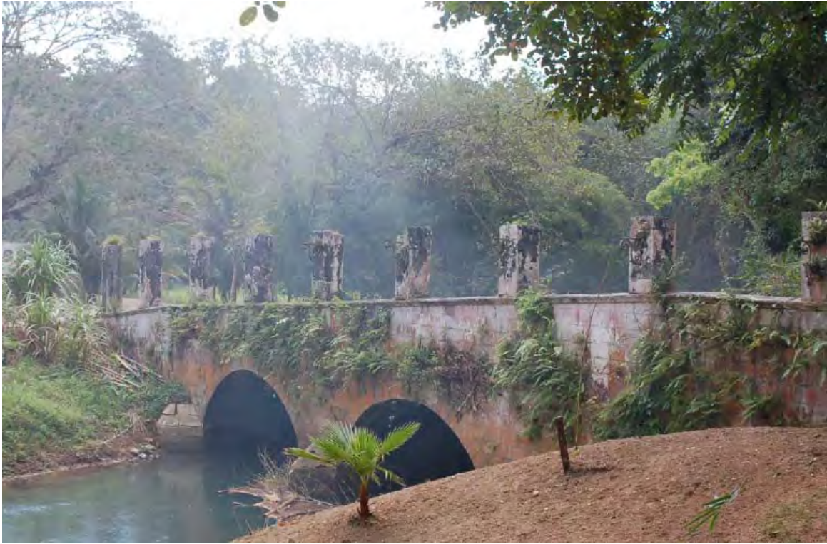
A mid-eighteenth century stone bridge at Good Hope Plantation spans the Martha Brae River. Iron brackets on the stone pillars once carried a trough that delivered raw cane juice from the wheel house to the processing complex. The smoke is from an early kiln reactivated to produce lime for restoration work.
