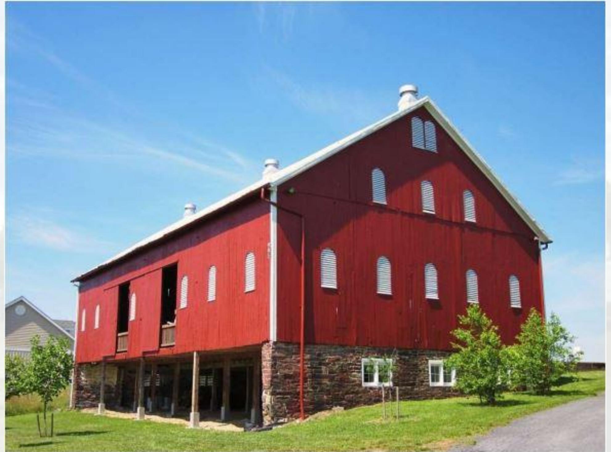
Bank Barn – Buckingham House and Industrial School Complex, past awardee, Frederick County
