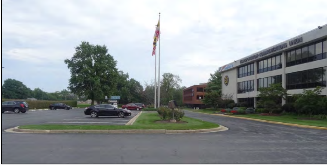
Figure 20: Washington National Pike Industrial Park.
