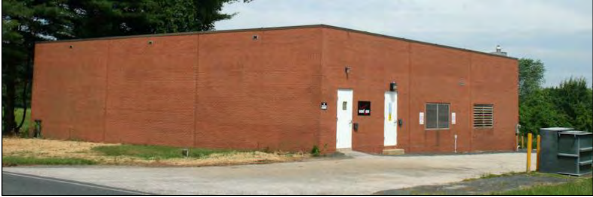
Figure 66: Telephone central office in Jarrettsville (1974).
