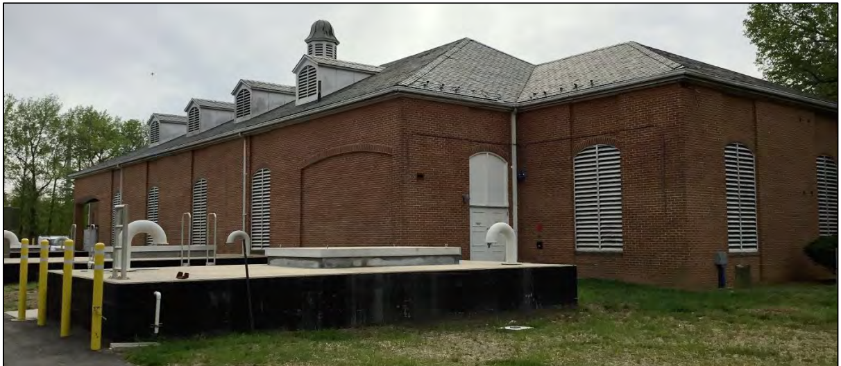
Figure 65: WSSC Central Avenue Water Pumping Station in Landover (1966-67).
