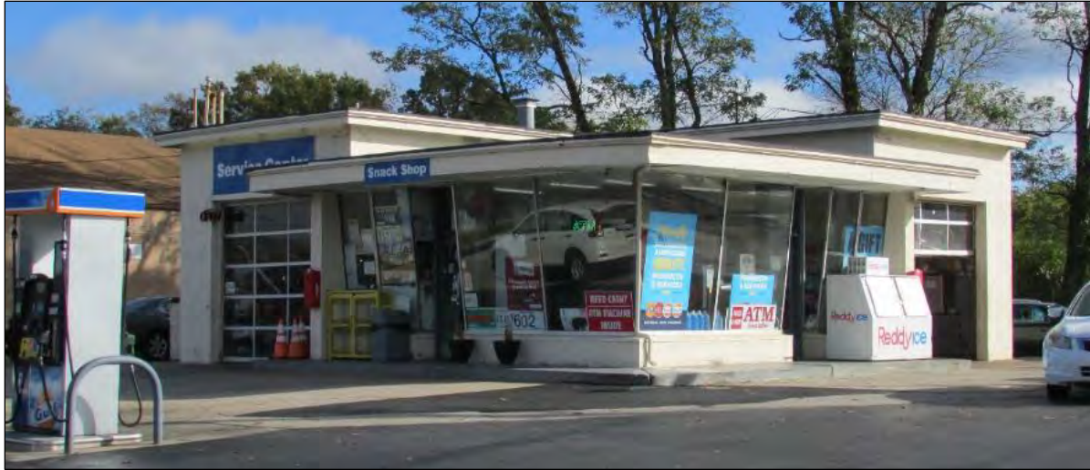
Figure 54: International Style gas and service station in Rockville (1963).
