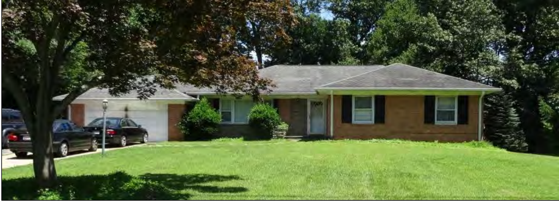
Figure 28: Example of a Ranch house in Colesville.
