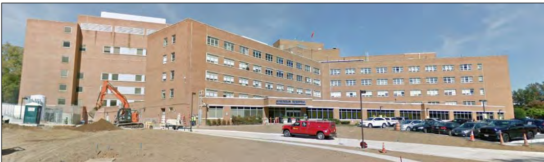
Figure 42: Modernist Suburban Hospital in Bethesda (1970).
