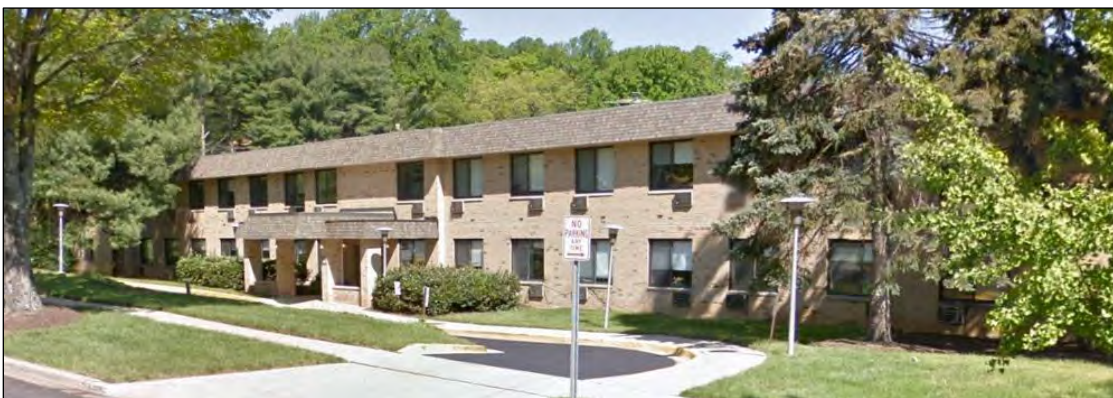
Figure 43: Collingswood Nursing Facilities in Gaithersburg (1972).
