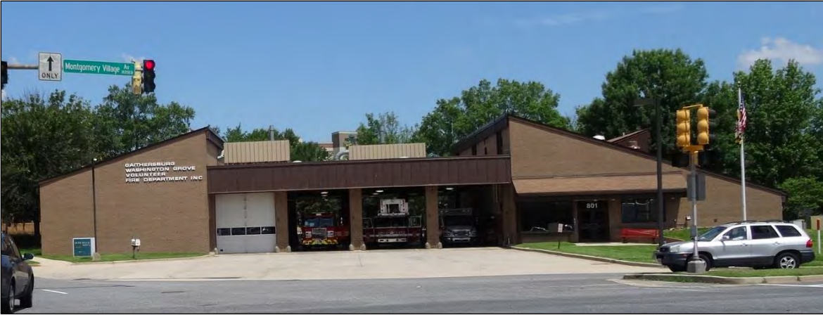
Figure 45: Shed-style Washington Grove Volunteer Fire Department, Station 8 in Gaithersburg (1975).
