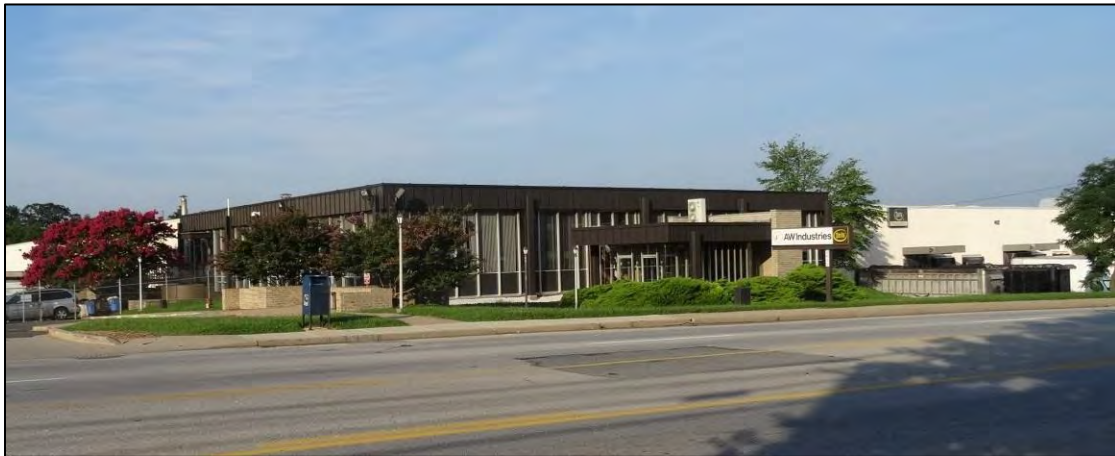
Figure 61: Serta Distribution Center and Offices in Prince George's County (1967).
