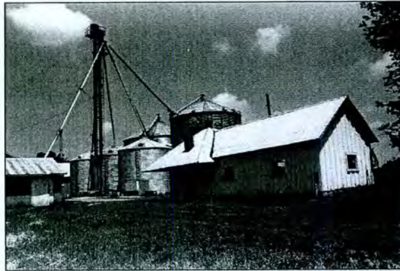
Figure 5-23: Rich Bottom (T-229) Smokehouse with Tool Shed to the Left
