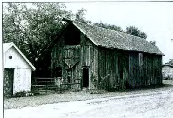
Figure 5-58: Country Rectory (T-387) Barn
