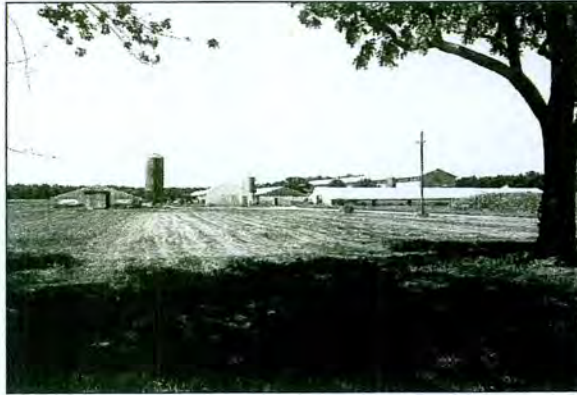
Figure 5-101: Poultry Farm at 30090 Lloyds Landing Road (T-392) Complex
