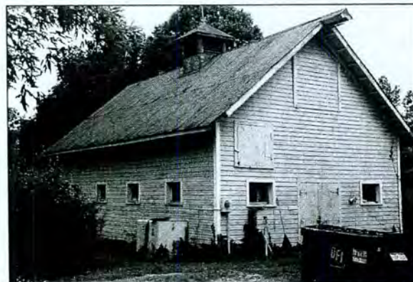
Figure 5-37: Chenar Farm (T-385) Dairy Barn
