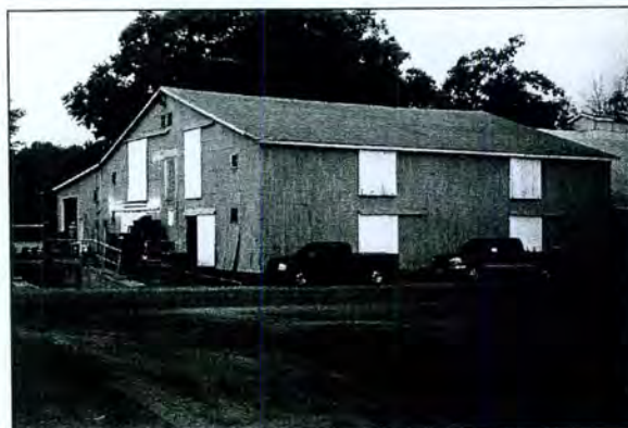
Figure 4-41: Defender Cannery (T-388) Cannery Building, constructed from ca. 1910 to ca. 1960
