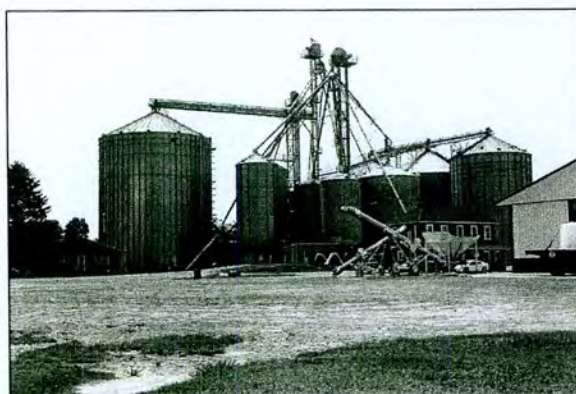
Figure 5-116: Wye Mills Feed Company (T-394) Grain Elevator and Grain Bins
