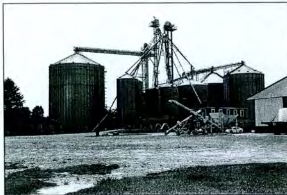
Figure 4-43: Wye Mills Feed Company (T-394) Grain Elevator and Grain Bins, constructed ca. 1974 to the present
