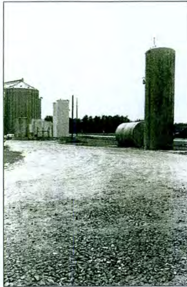
Figure 5-117: Wye Mills Feed Company (T-394) Fertilizer Tanks
