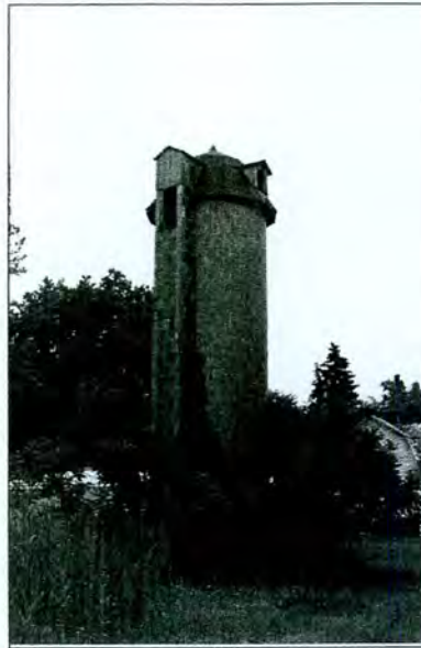
Figure 5-39: Chenar Farm (T-385) Silo
