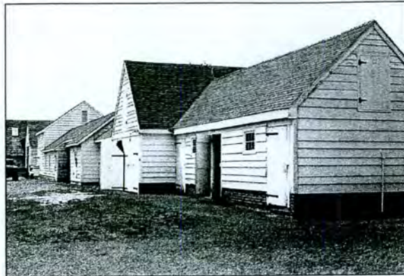
Figure 5-17: Langdon (T-215) Outbuilding Block
