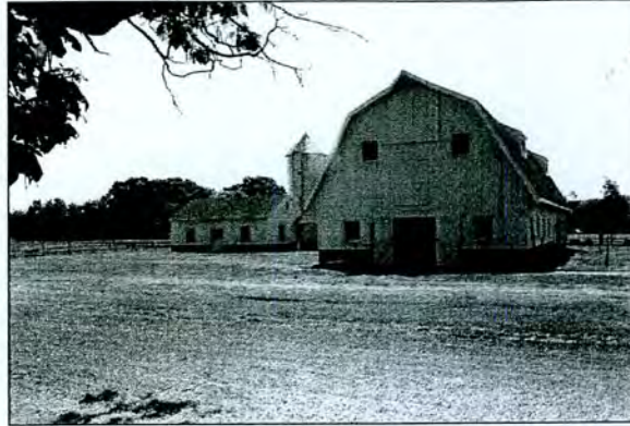
Figure 5-1: Radcliffe Manor (T-42) Dairy Complex
