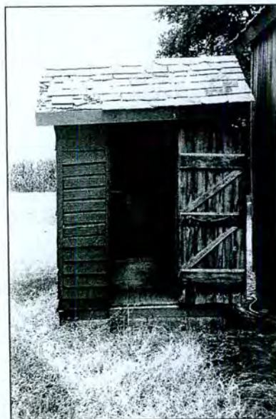
Figure 4-11: Clarke W. Sewell Farm (T-393) Wood Frame Privy, constructed ca. 1920
