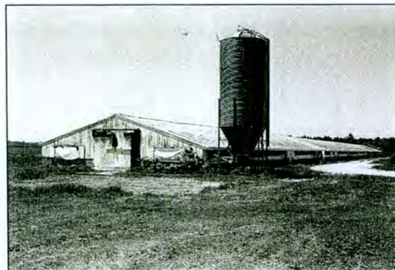
Figure 5-104: Poultry Farm (T-392) Broiler House #1 with Grain Bin
