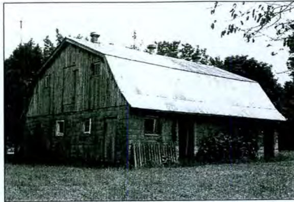
Figure 5-28: Schofield House (T-342) Barn
