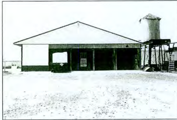
Figure 5-121: Wye Mills Feed Company (T-394) Second Timber Frame Warehouse
