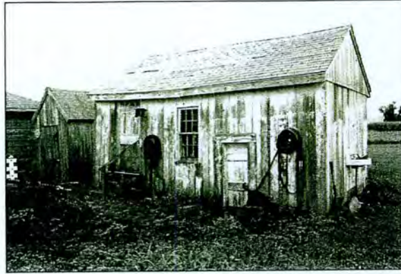
Figure 5-127: Voshell Farm (T-395) Smokehouse (left) and Pump House (right)
