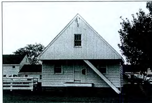
Figure 5-16: Langdon (T-215) Storage Building
