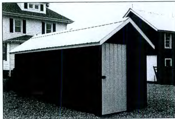
Figure 4-12: Mullikin Farm (T-389) Pump House, constructed ca. 1915
