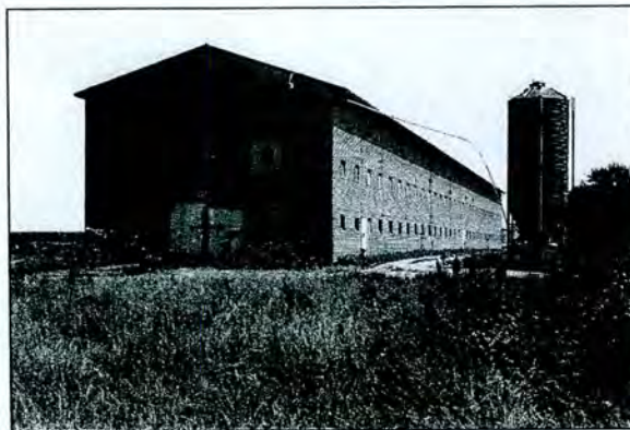
Figure 4-39: Poultry Farm at 30090 Lloyds Landing Road (T-392) Hatchery, constructed ca. 1960
