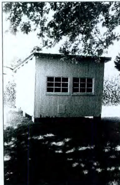
Figure 4-35: Lindemann Farm (T-391) Hen House, constructed ca. 1937
