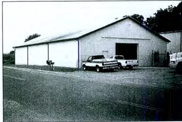
Figure 4-42: Defender Cannery (T-388) Warehouse, constructed ca. 1935
