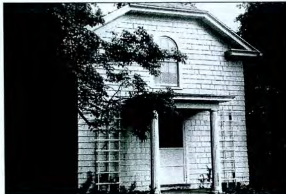
Figure 5-36: Chenar Farm (T-385) Powerhouse
