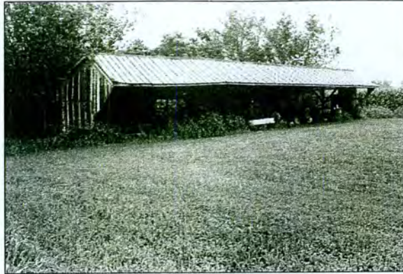
Figure 5-129: Voshell Farm (T-395) Machinery Shed
