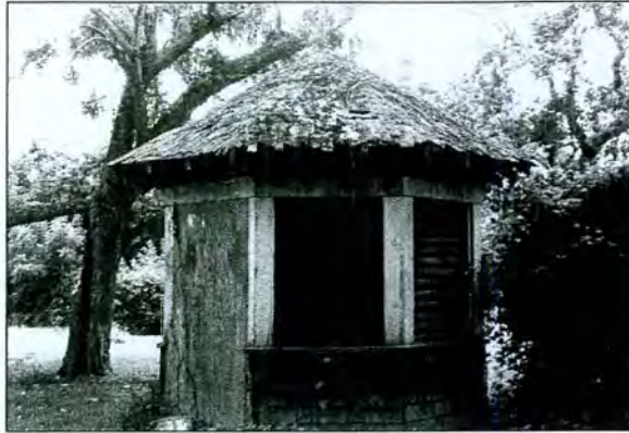
Figure 5-41: Chenar Farm (T-385) Gas House
