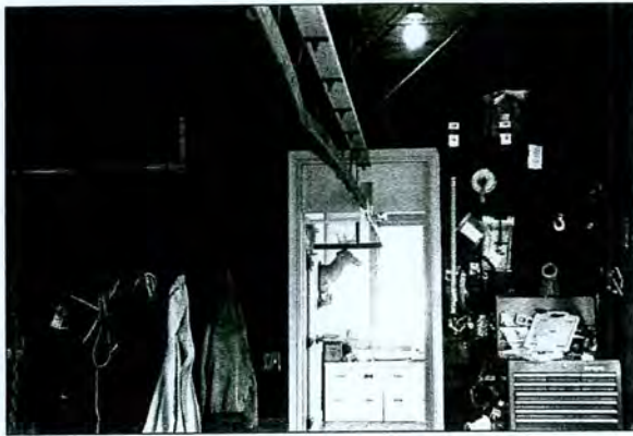
Figure 5-14: Steel Meat Rail in Langdon (T-215) Slaughterhouse (left)
