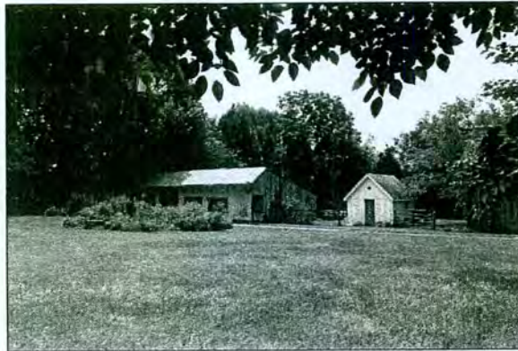
Figure 5-57: Country Rectory (T-387) Carriage House (left) and ca. 1950 Milk House (right)
