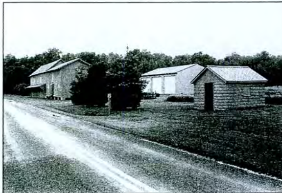
Figure 5-45: Cottingham Farm Orchard Buildings (T-386) Complex
