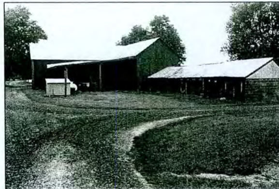
Figure 5-111: Clarke W. Sewell Farm (T-393) Barn with Machine Shed Addition
