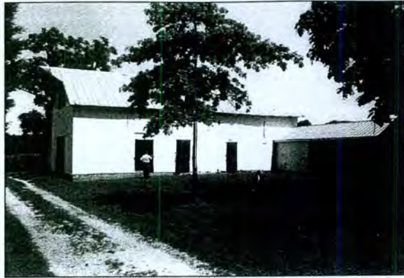
Figure 4-18: Lindemann Farm (T-391) Barn with a Hay Hood, constructed ca. 1900
