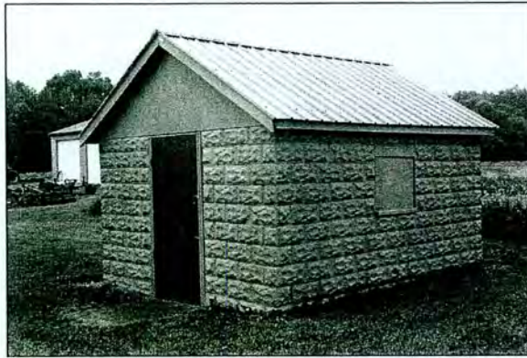
Figure 5-48: Cottingham Farm Orchard Buildings (T-386) Masonry Shed
