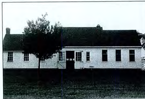
Figure 5-13: Langdon (T-215) Slaughterhouse
