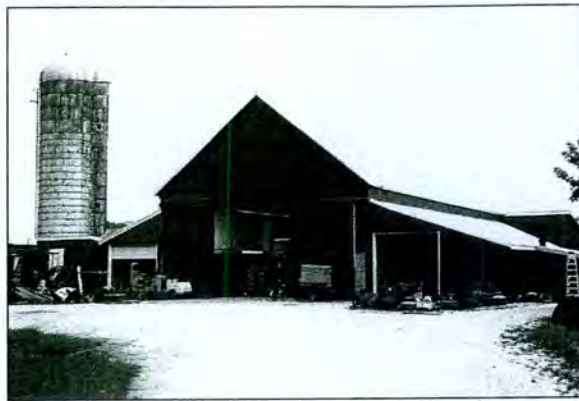
Figure 4-17: Mullikin Tenant Farm (T-390) Gable Roof Barn with Side Shed Roof Additions, constructed ca. 1910
