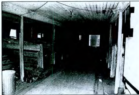
Figure 4-22: Radcliffe Manor (T-42) Dairy Barn Interior with Stalls, a Concrete Floor, and Drainage Channels, constructed ca. 1935
