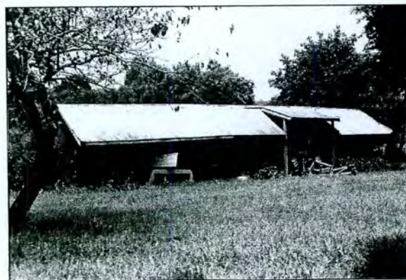
Figure 5-29: Schofield House (T-342) Machinery Shed
