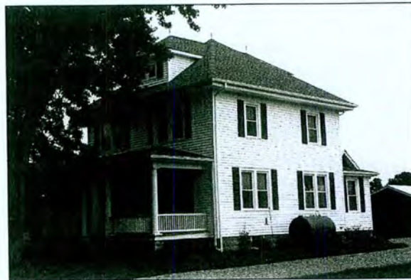
Figure 5-74: Mullikin Farm (T-389) Residence
