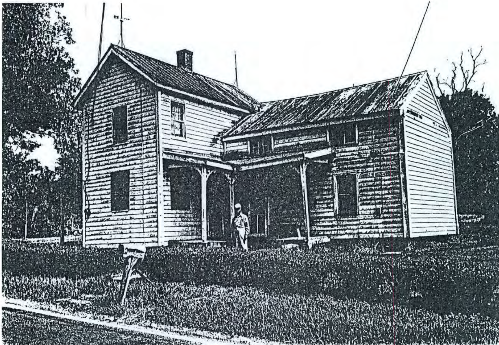
Figure 60. Albert Thompson house, Martinsburg. John Thompson is standing in front of the original log house of his grandfather, Albert Thompson. It is the one and a half story block at right (c. 1877). It was covered with weatherboards in 1916, when John's father, Otho Thompson, added the frame section at left.
