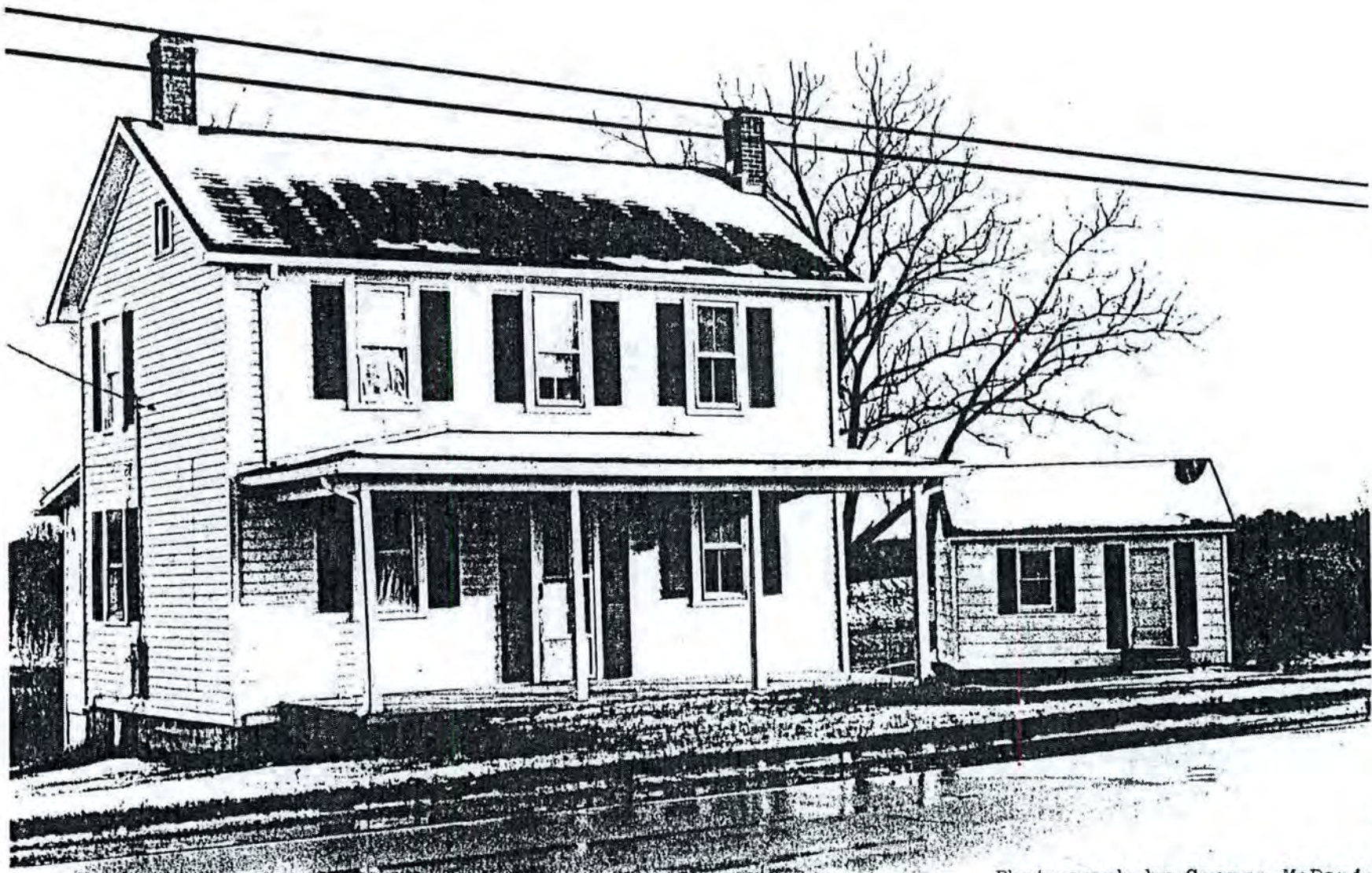
Figure 12. Arthur Gibson House, Clarksburg. This two story house was built in c. 1918 by the black carpenter, Arthur Gibson, and renovated by Gibson's nephew and namesake, Arthur Randolph. It is perhaps the best preserved of the houses built by black carpenters in the survey area.
