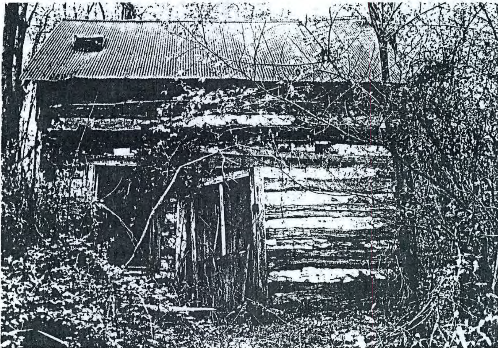
Figure 49. Frank Dorsey log house, Jerusalem. With one room down and one up, and a frame shed kitchen on the back length, this house was smaller than most. Like other log houses of black families in the survey area, this one will soon collapse, leaving little trace of its existence above ground.
