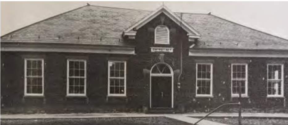
Figure 10. The 1909 Greensburg School in Washington County, a Colonial Revival-style brick building with a slate roof, had three classrooms for 90 students in grades one to six and a kitchen. Washington County reused and adapted this plan and exterior treatment for several schools built there from the 1910s through the 1930s. 70
