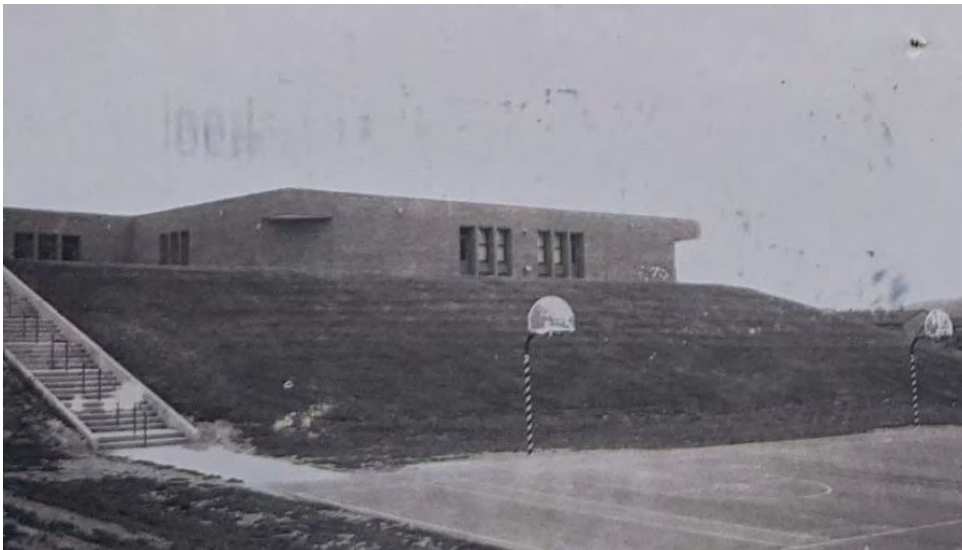
Figure 87. Gwynn Park Senior High School in Charles County (1975 addition; top), Edgewood Senior High School in Harford County (ca. 1970 addition; middle), and South Lake Elementary School in Montgomery County (1972; bottom) are examples of Late Modern architecture. 401
