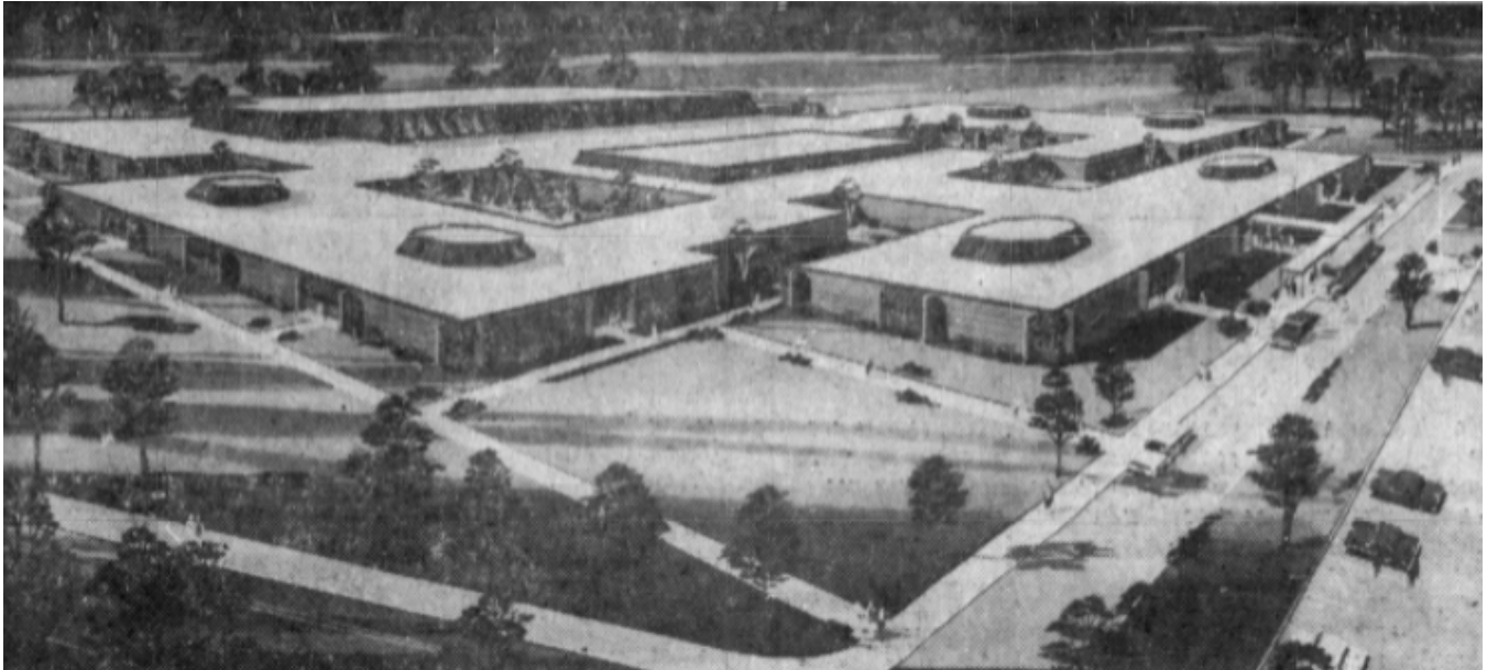
Figure 76. Sykesville Elementary School in Carroll County (1970), designed with five pod-like clusters of four classrooms each, with a central shared commons area. 390
