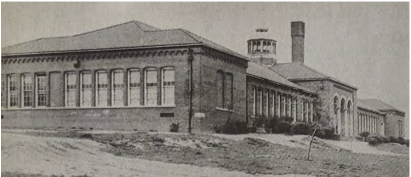
Figure 20. The 1926 Benjamin Franklin High School in Baltimore City was designed in the Renaissance Revival style with an arched entry, arched window openings, a ceramic tile roof, and stylized arched denticulation at the cornice. 123
