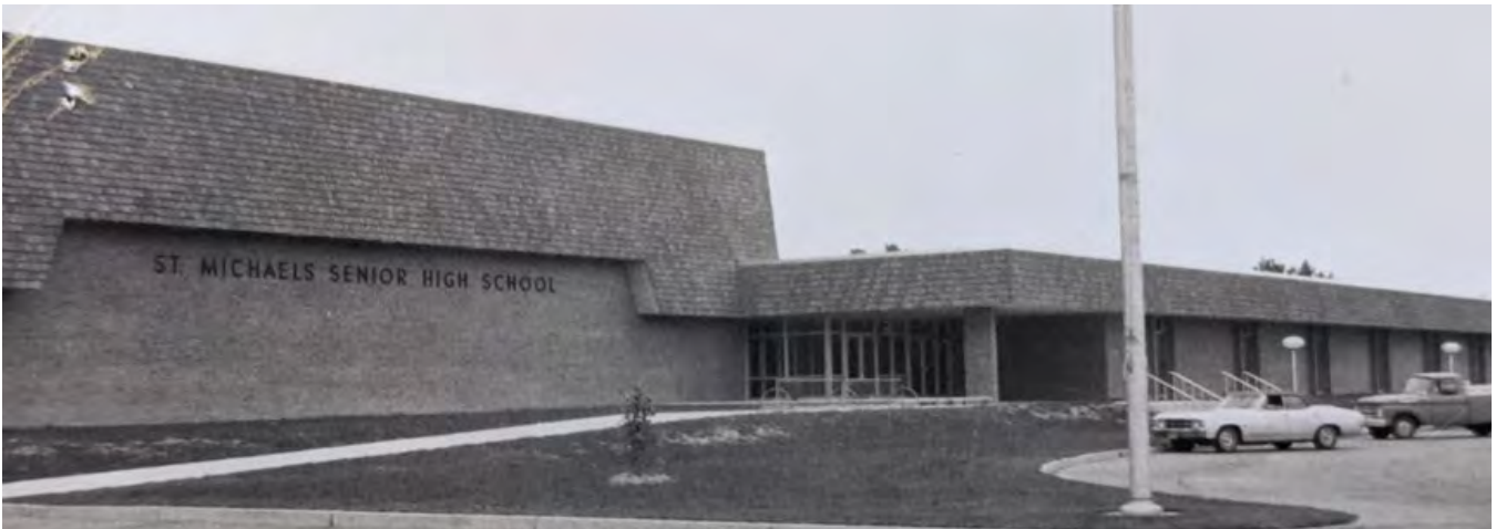
Figure 84. Mansard roof volumes within flat-roof sections of Barton Elementary School (1975; top) and Eldersburg Elementary School in Carroll County (1970; middle). Shingled mansard roof at St. Michael's Senior High School in Talbot County (1971; bottom). 398
