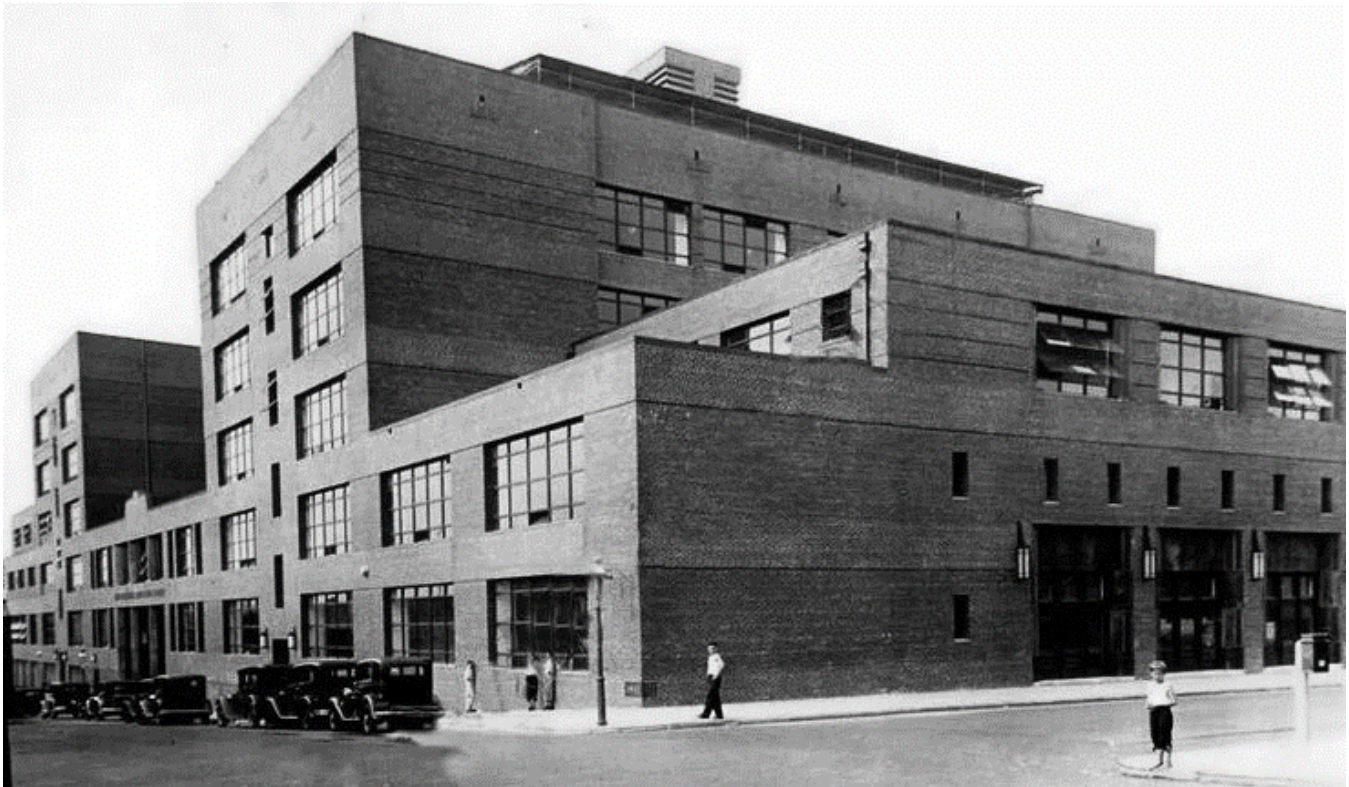
Figure 35. The 1934 Patterson Park Senior-Junior High School in Baltimore City was one of the most important examples of Early Modern-style school architecture in the state. 174
