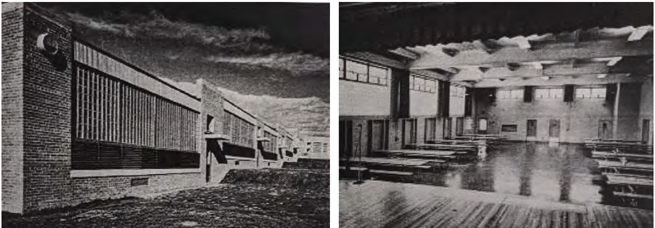
Figure 64. Fountaindale Elementary School, a model elementary school designed by Rhees Burket in collaboration with educational consultant Nicholas Engelhart, had light-filtering glass block windows and classrooms that opened to the outside to facilitate indoor-outdoor teaching (left). Each classroom had its own terrace and garden plot. Interiors were thoughtfully designed with flexible, space-saving features, such as the tables that folded up into the walls in the combination cafeteria-gymnasium, both in Washington County (right). 308
