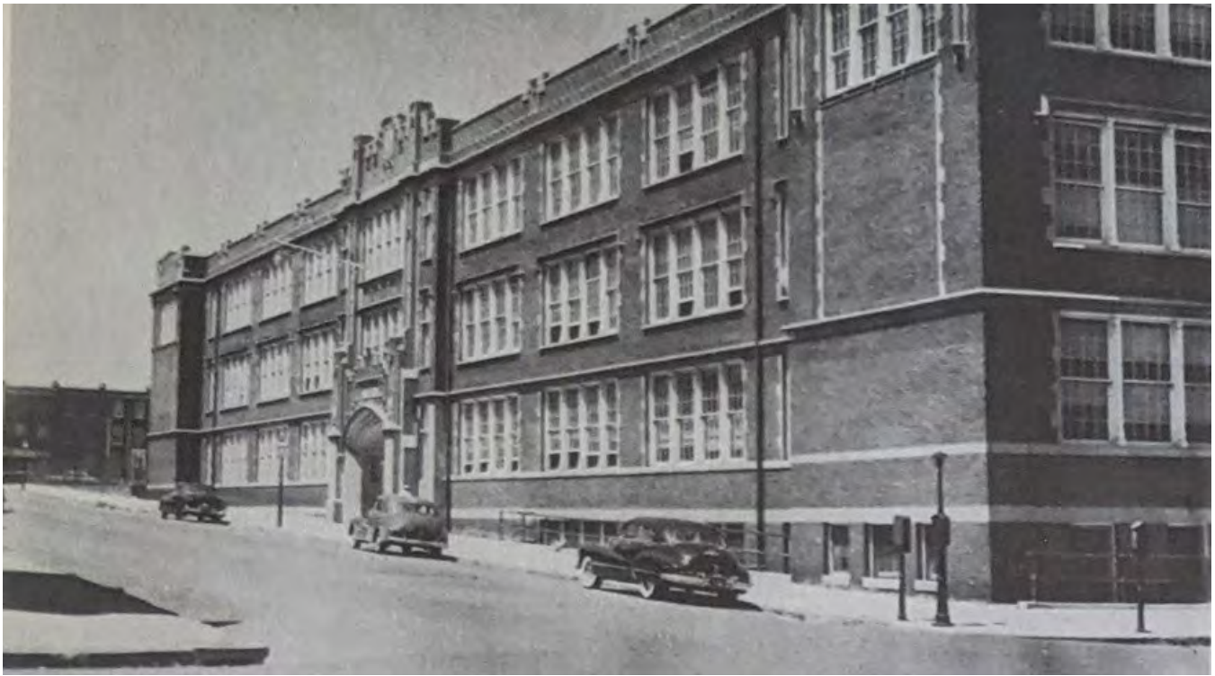
Figure 15. Built in 1924, the third rendition of the Frederick Douglass Junior-Senior High School in the Sandtown-Winchester neighborhood of Baltimore City was the first public high school built specifically for Black students in Maryland. It was constructed as part of the city's efforts to improve school facilities deemed inadequate by the 1921 Strayer report. 103
