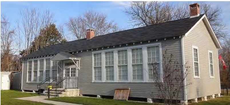
Figure 100. A renovated ca. 1926 Rosenwald School, Galesville, Anne Arundel County, in 2012. 441
