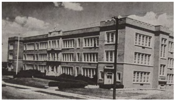
Figure 115. Westport Elementary School, built in 1924, Baltimore City, in the 1950s. 470
