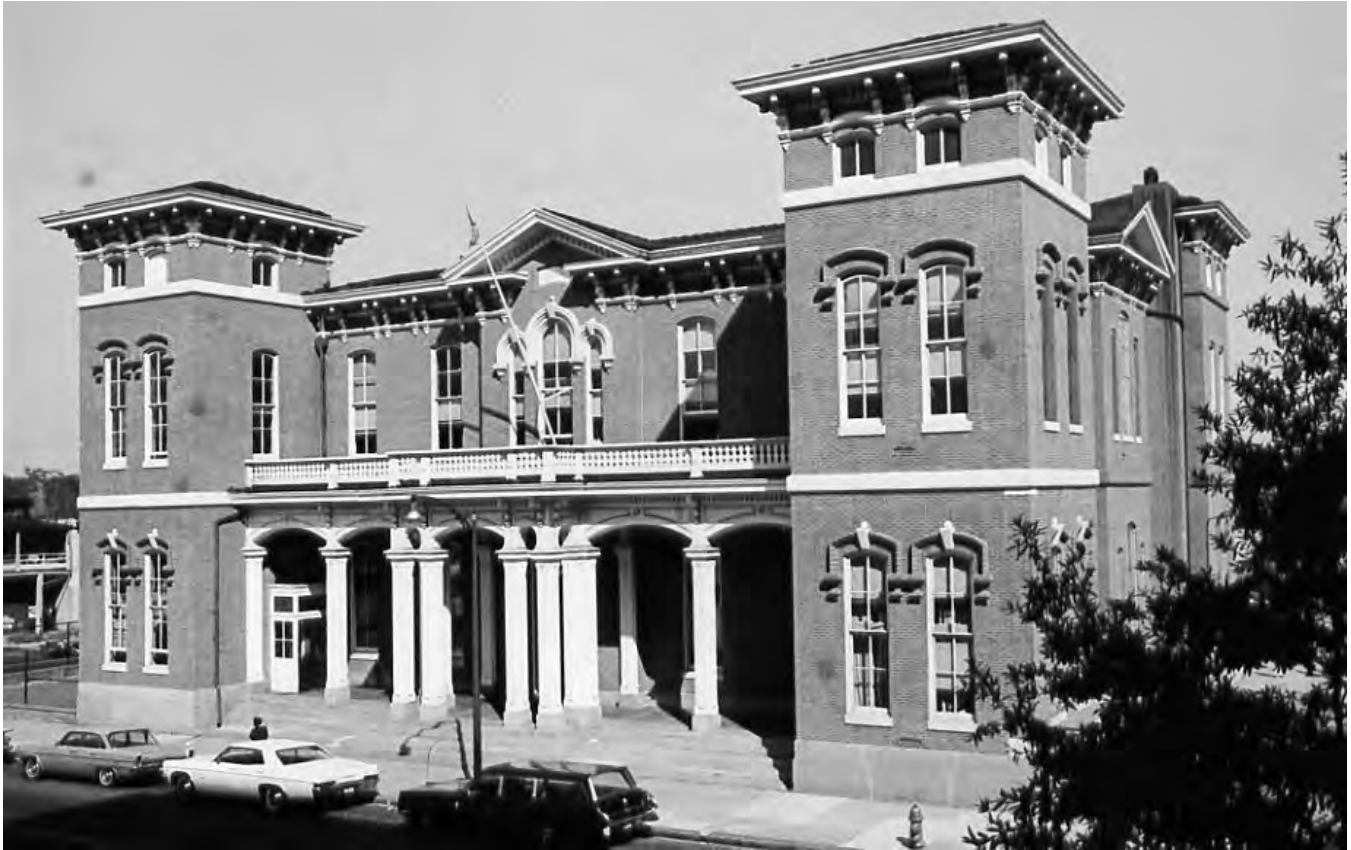
Figure 6. Noted architect Colonel R. Snowden Andrews designed the 1870 Eastern Female High School in Baltimore City. In 1850, Baltimore became the first city in the country to establish public high schools for girls: Eastern Female High School and Western Female High School. Permanent facilities that prominent architects designed were constructed in 1870. 57
