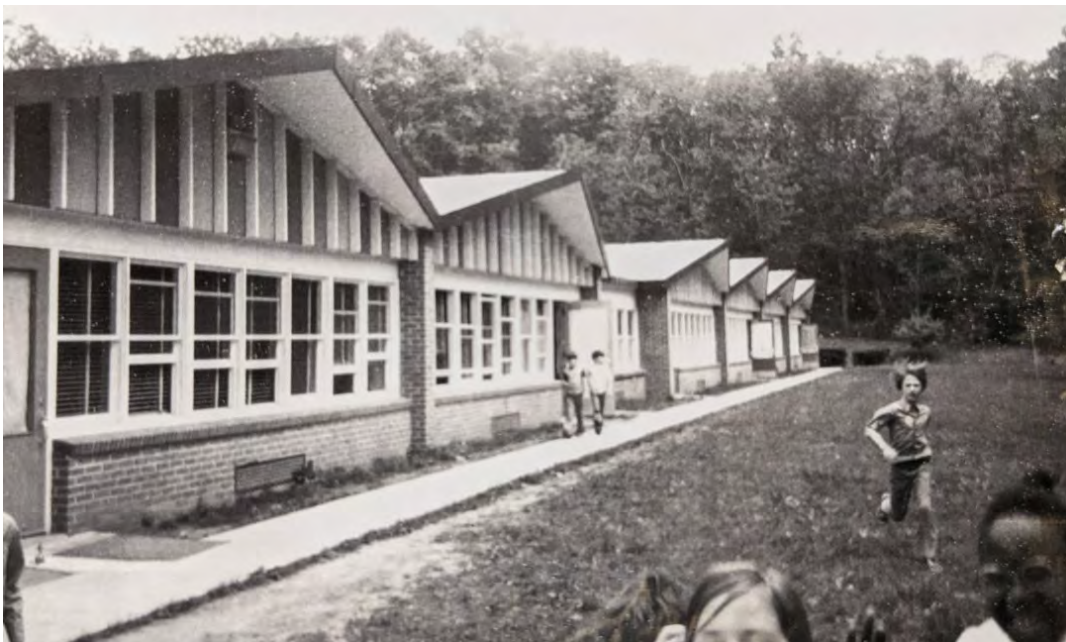
Figure 81. Manor View Elementary School (1971; top), a design repeated for at least five other Anne Arundel County Schools in the late post-World War II period. Colonel Richardson Junior High School in Caroline County (middle) and Cascade School addition in Washington County (1965; bottom). 395
