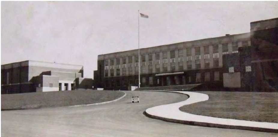
Figure 39. The Art Deco-style Fort Hill School in Allegany County, was completed in 1936 with PWA funding. 180
