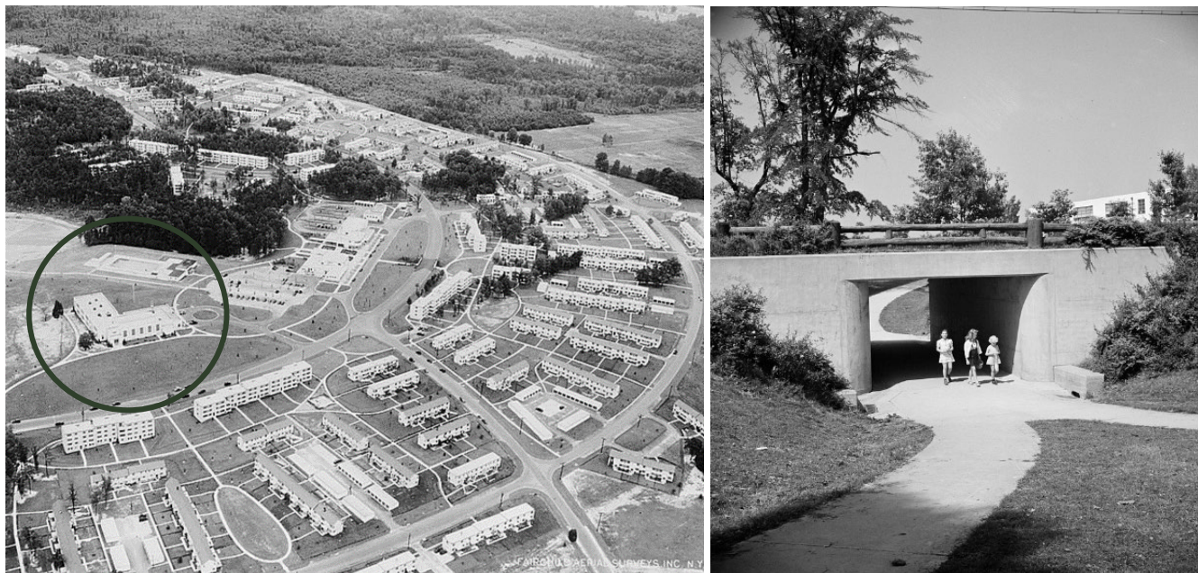
Figure 29. In Greenbelt, Prince George's County, an early and experimental master-planned community, the school (circled, left) was placed at the neighborhood's geographic and social core. The building, which was within walking distance from all homes and public spaces via a network of pedestrian paths with underpasses below busy roads so children could walk to school safely (right), was also adjacent to a park and woodlands that were used for recreation and hands-on learning in nature. With dual-purpose spaces, the school could be used for community functions outside of school hours. 160
