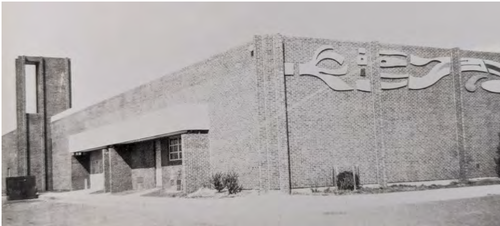
Figure 139. Coldstream Park Elementary School #31, built in 1970, by Rogers and Vaeth, Baltimore City. Façade sculpture by Earl Hofmann. The pierced tower is a clear Late Modern-style homage to the influential Early Modern-style 1940 Crow Island School. 512
