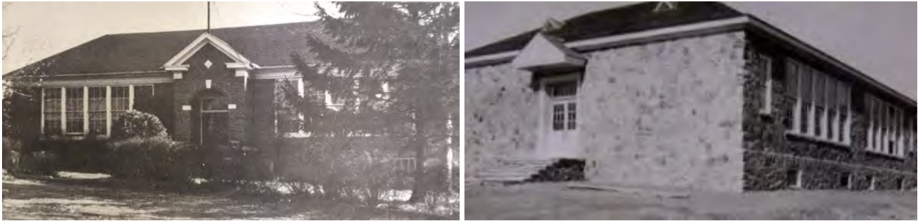
Figure 31. These 1930s rural elementary schools were designed with Maryland's traditional aesthetic. The 1931 Big Pool Elementary School (left) in Washington County is based on the ubiquitous Colonial Revival-style that the county had employed since the 1910s. The 1939 Port Deposit Colored School in Cecil County was a stone building completed with WPA funds (right). 168
