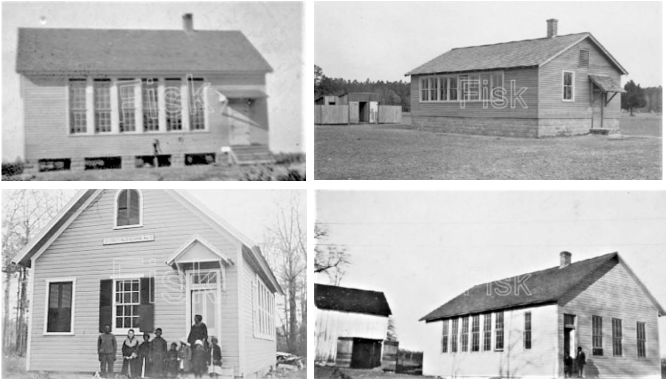
Figure 18. Natural light streamed through bands of tall windows along these one-teacher one-room Rosenwald schools. Of wood-frame construction with gable roofs, each had a chimney, water pump, and outhouse. Clockwise, from upper left, are the Bishop School in Worcester County, Jonestown School in Caroline County, Swan Creek School in Harford County, and Island Creek Neck School in Talbot County. 116
