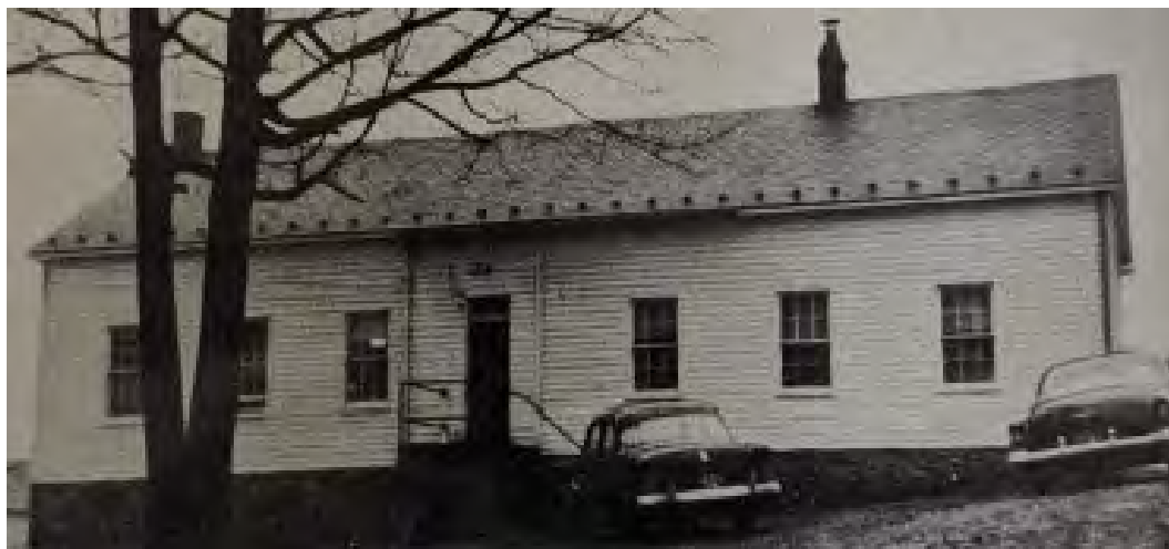
Figure 8. The 1882 Yarrowsburg School in Washington County is a typical two-room, wood-frame schoolhouse. The building had capacity for 60 students in grades one to six, outdoor toilets, and a coal stove for heat. 63
