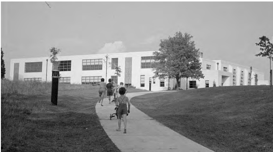
Figure 40. Greenbelt's 1937 Center Elementary School was a groundbreaking example of Modernism in Maryland. 181
