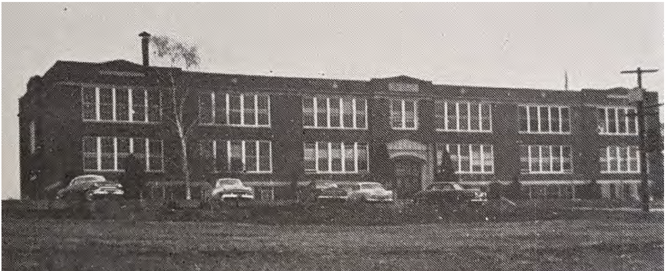
Figure 22. Washington County's 1926 Boonsboro High School is a typical 1920s rural high school in Maryland. Its architectural treatment was minimized to the accentuated central entrance and symmetrically placed banks of windows that provided natural light and fresh air. 126
