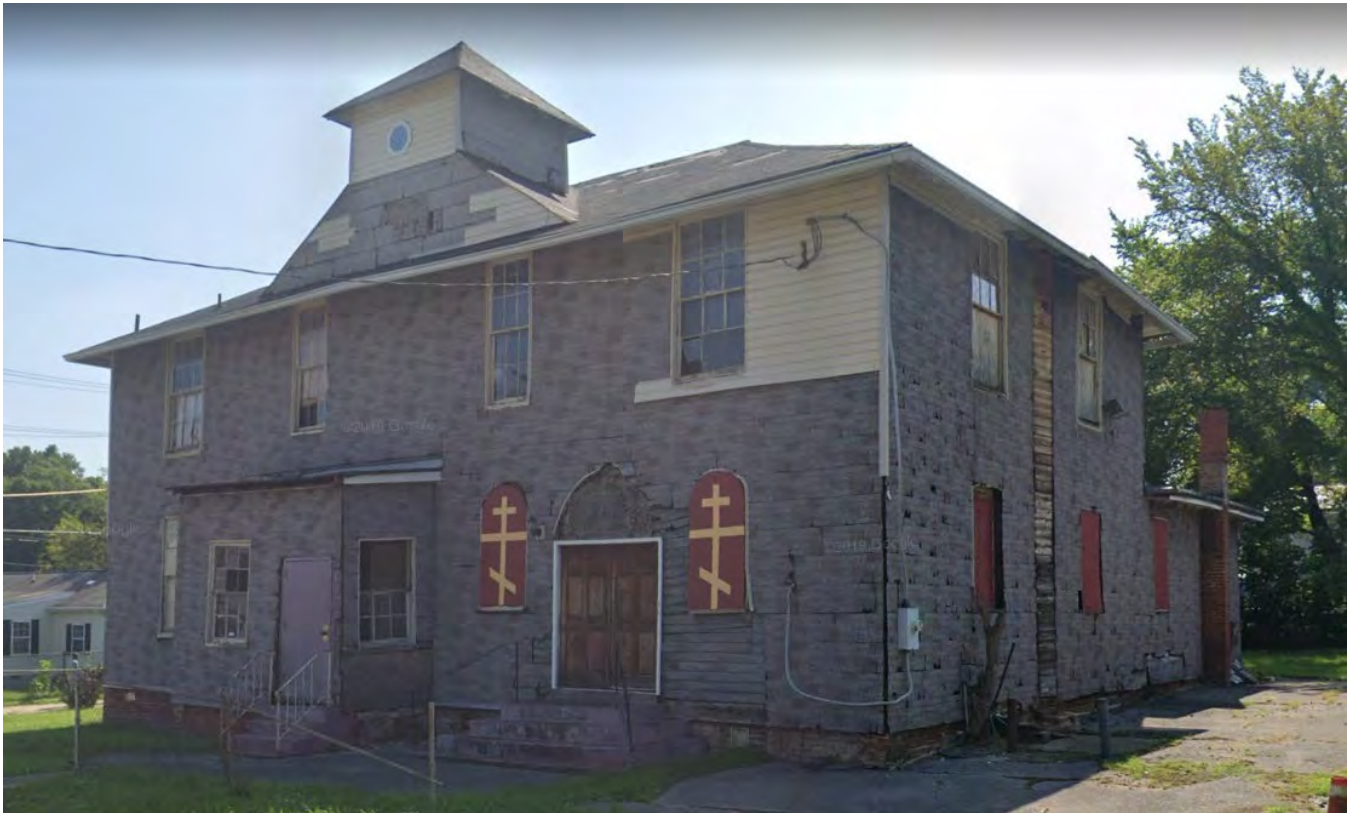
Figure 144. The 1912 Fairmount Heights Elementary School was an integral part of Fairmount Heights, a planned suburban community for Black residents, and it was the first school for Black students in Prince George's County. It is a rare known example of a Maryland school designed by a Black architect, and one of William Sidney Pittman's last designs in the state. 528 The highly significant building is listed in the NRHP as contributing to the Fairmount Heights District and is a strong candidate for preservation and restoration. 529
