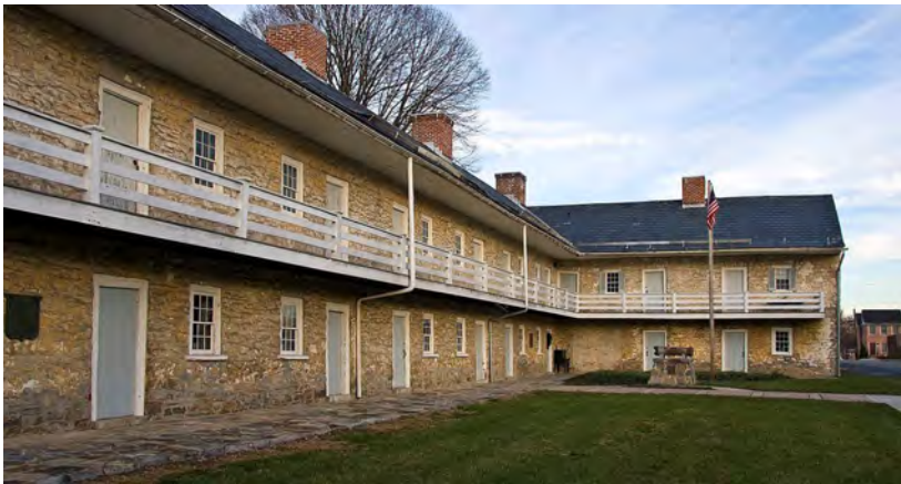
Figure 5. The extant Hessian Barracks building at the Maryland School for the Deaf (Frederick County). 52
