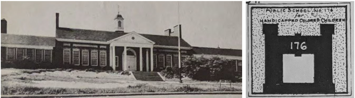
Figure 30. The front façade (left) and footprint (right) of the 1933 Francis M. Wood School in Baltimore City, a school for disabled Black children, combined traditional architectural stylistic influences with the more-modern courtyard plan. The courtyard reduced travel time between wings and safely separated play space from vehicular traffic. Other modern planning provisions were extra-wide doorways and hallways, facilities for physical therapy and other treatments, special lighting and furniture for the visually impaired, and rooms with specially designed floors that vibrated to help deaf children develop a sense of rhythm to improve their speech. 167
