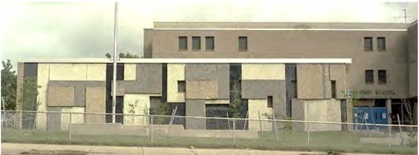
Figure 88. Brutalist-style John Humbird Elementary School in Allegany County (1974; top) and Westside Elementary School in Baltimore City designed by notable Black architecture firm Fry and Welch (1973; bottom). 402 Located in the historically Black neighborhood of Mondawmin in West Baltimore City, Westside Elementary School included an outdoor teaching space between the playground and school. 403
