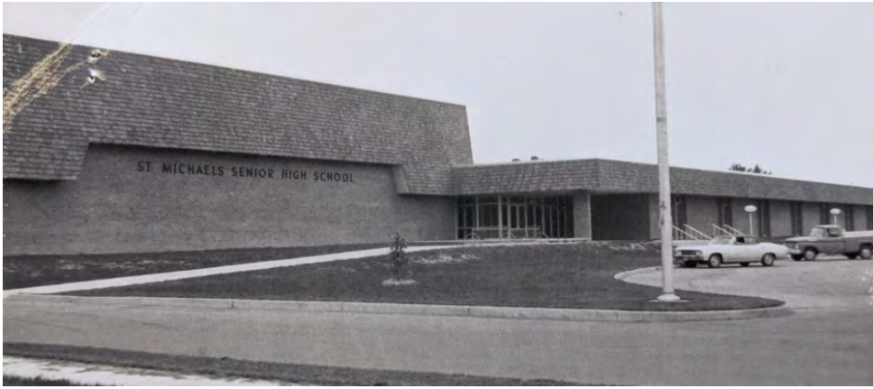
Figure 141. St. Michaels Senior High School, built in 1970, by Buchart Associates, St. Michaels, Talbot County; undated photograph. 514
