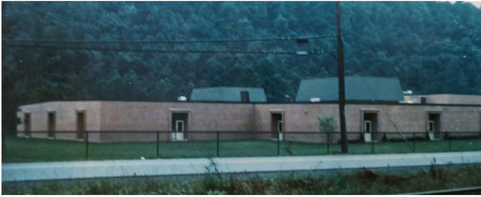
Figure 138. South George's Creek Elementary School, built in 1973, by Johannes & Murray Associates, Lonaconing, Allegany County, in 1976. 511
