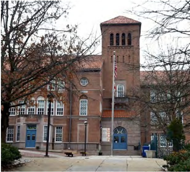
Figure 117. Roland Park Elementary/Middle School, built in 1925, by P. C. Street Engineering Company, Baltimore City, in 2020. 474
