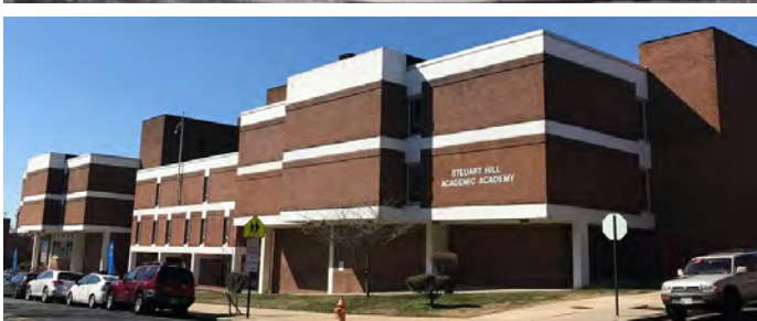
Figure 137. Stuart Hill Elementary School #4, built in 1969, by Tatar and Kelly, Baltimore City, in 2018. 508
