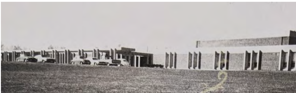
Figure 140. Havre de Grace Middle School, built in 1967, Havre de Grace, Harford County; undated photograph. 513
