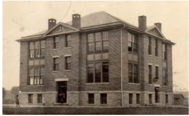
Figure 102. North East High School, built ca. 1898, Cecil County, in the 1910s. 445
