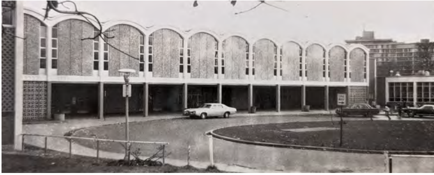
Figure 130. Albert Einstein Senior High School, built in 1962, Kensington, Montgomery County, in the 1970s. 497
