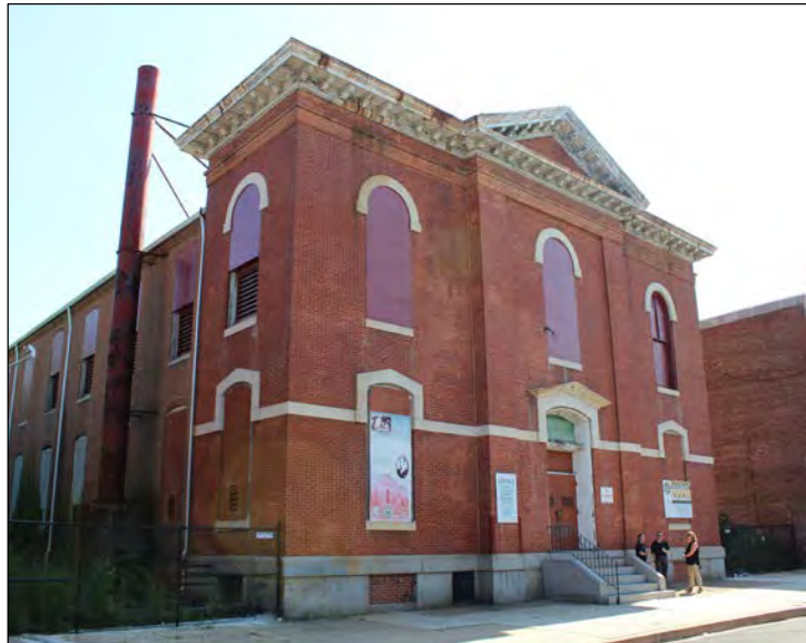
Figure 1. Public School 103 (EHT Traceries, 2015)
