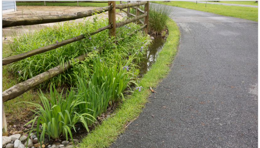
Figure 3.10 - Zoning requirements can include limiting stormwater run-off through the use of drainage ditches and rain gardens. Shadyside, Anne Arundel County.
