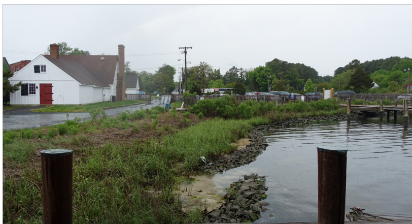
Figure 3.5 - Natural shoreline protection of marsh infill behind small rocks to protect historic buildings. St. Michaels, Talbot County.
