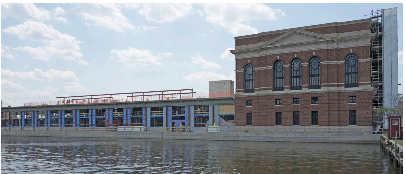
Figure 3.20 - Dry floodproofing is hidden behind the building's façade at the Recreation Pier. Fells Point, Baltimore City.
