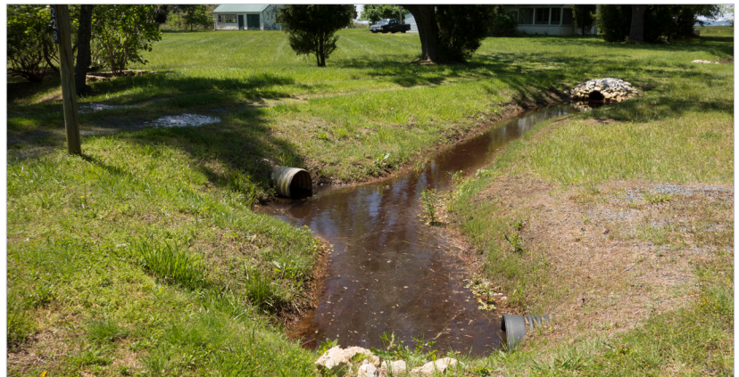
Figure 3.8 - Engineered drainage system to convey stormwater to a retention area away from historic cottages. Shady Side, Anne Arundel County.
