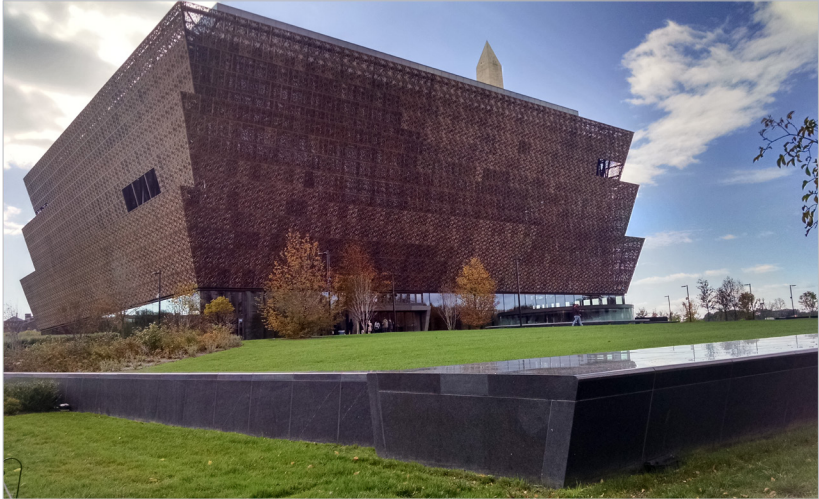
Figure 3.23 - Flood wall (black granite, foreground) forms a perimeter barrier surrounding the National Museum of African American History and Culture and protects the museum from flooding by the Potomac River. Washington, DC.
