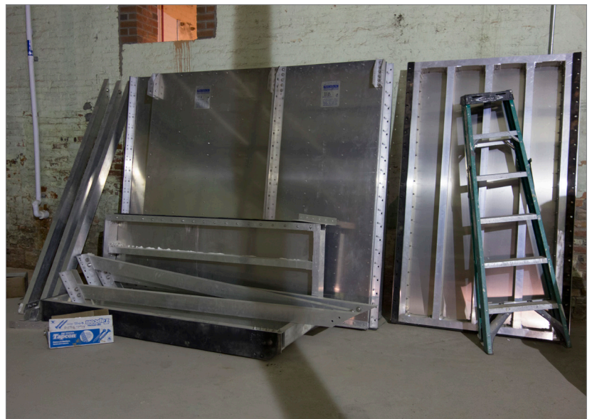
Figure 3.21 - Metal flood barriers for covering exterior doors are stored inside the Mount Vernon Mill #1, Baltimore City.
