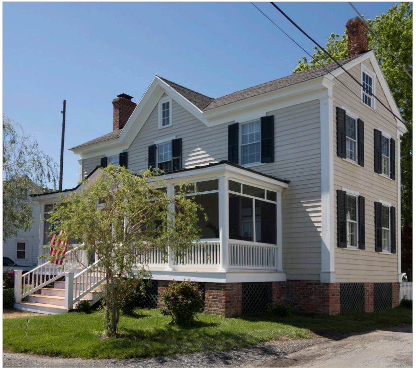
Figure 3.17 - Sensitive elevation of historic building. Whitehaven, Wicomico County.
