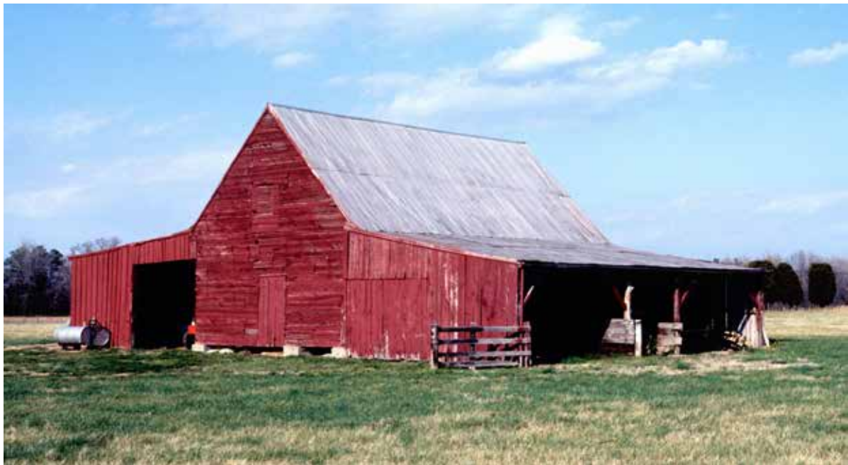
In 2007, Non-Capital Program funds supported documentation of Southern Maryland tobacco barns with photographs and measured drawings. These barns, a defining feature of the agricultural landscape for hundreds of years, are rapidly disappearing. The Brome Howard Barn, pictured here, is located in St. Mary's County and dates to 1785.
