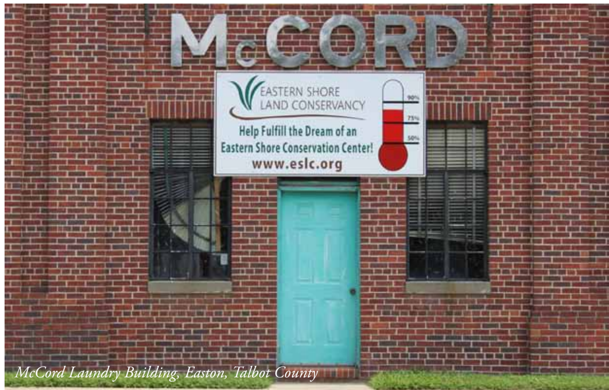
The former McCord Laundry is now home to the Eastern Shore Land Conservancy, Chesapeake Bay Foundation, Ducks Unlimited, The Nature Conservancy, and Town Creek Foundation. The project utilized State bond bill funds, which resulted in an easement, and rehabilitation tax credits.
